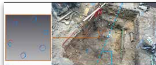
Horizontal cut of the rebars showing accurate comparison of photogrammetry to terrestrial laser scanning (TLS): blue circles represent photogrammetry, and red circles represent TLS; maximum deviation is ~6-10 millimeters.
