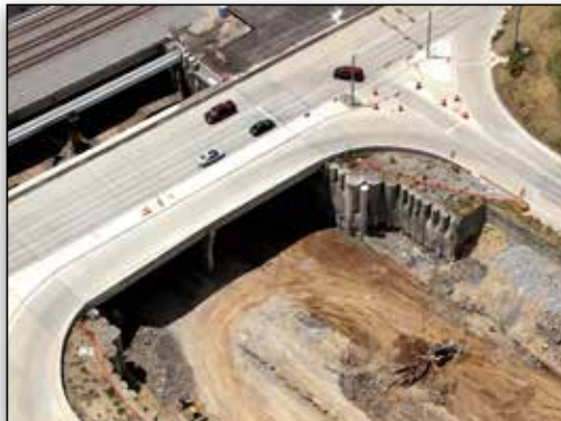
An aerial view of the Texas State Highway 161 under construction.
