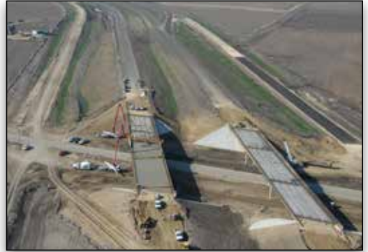
View of Texas State Highway 130.
