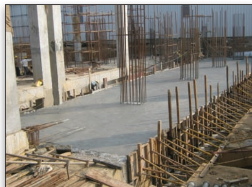
Mat foundation ready for formwork to be removed
