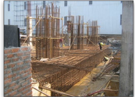
Six feet deep mat foundation rebar cage ready for concrete pouring
