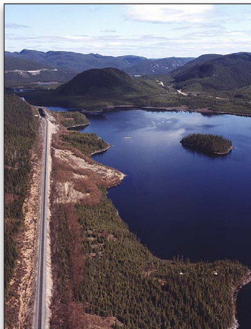
ArcelorMittal Mines railroad spans over 250 miles in Québec, Canada.
