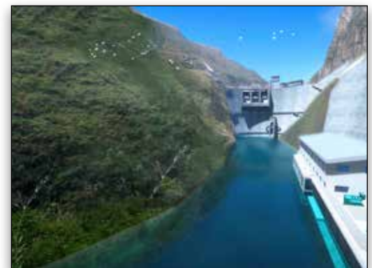
The project model created in MicroStation accurately reflected the complex environmental conditions of the region and provided a solid foundation for the overall 3D design.
