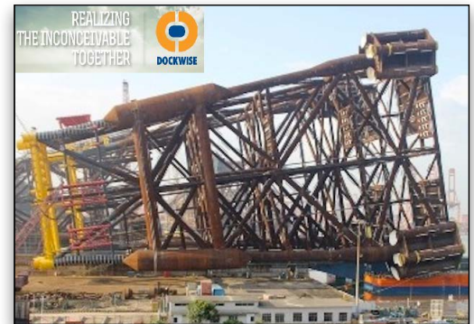
SHWE Jacket Load-out.
