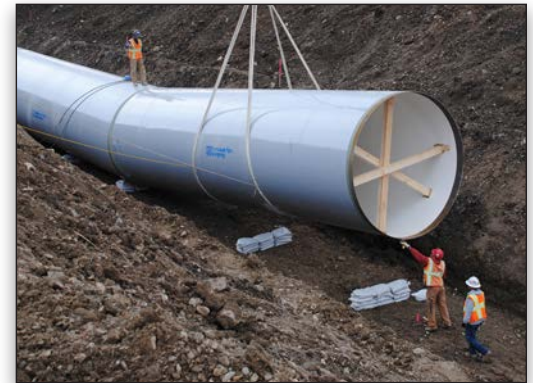
Workers installing the 126-inch diameter buried pipeline.
