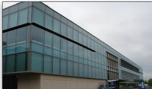
Flad Fill-Finish South Facade
