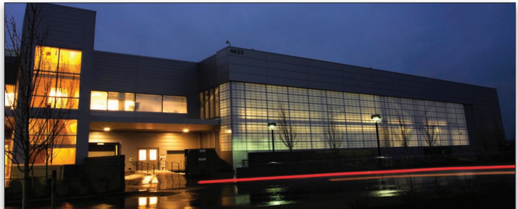
Flad Fill-Finish East Facade
