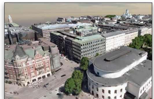
Helsinki used Bentley applications to create a reality mesh and a CityGML intelligent model of the city.
