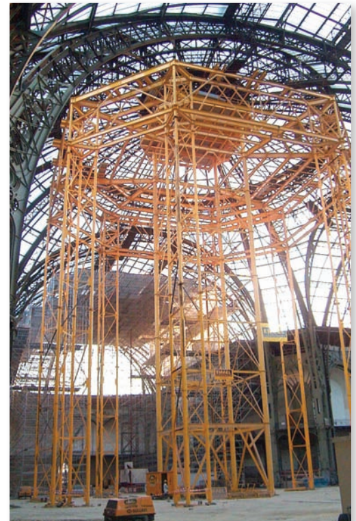
Project included renovation of the metal framework and glass canopies
