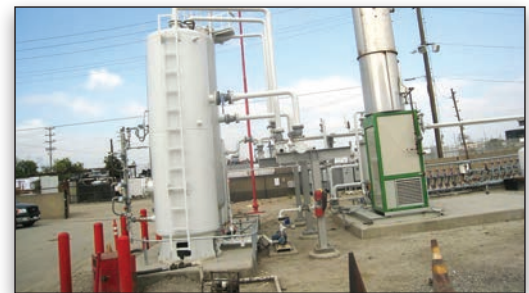
A rendering of a vertical vessel with foundation designed in a confined space.
