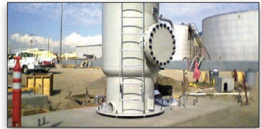
This image captures the 4-foot diameter vessel after installation.
