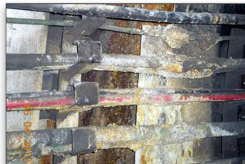
*Original tunnel lining installed in the 1970s showed signs of water ingress, causing potentially unsafe conditions.*
