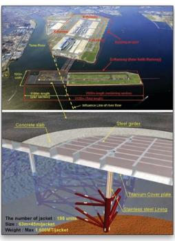
NSENGI built an offshore runway at Tokyo International Airport, using SACS to design the jacket-supported pier structure. Image courtesy of Joint Venture Group for D-Runway Construction in Tokyo International Airport (Haneda Airport) Re-expansion Project.
