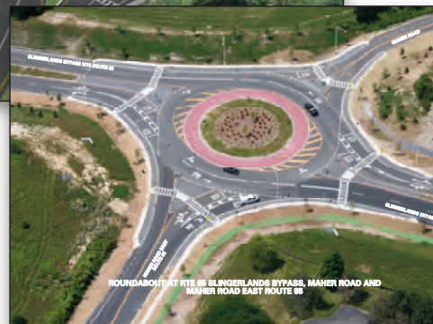
Three two-lane roundabouts replaced signalized intersections to improve safety
