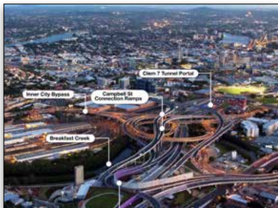
The project consisted of two tunnels, a new airport connection and involved 6.7 kilometers of underground toll roads.
