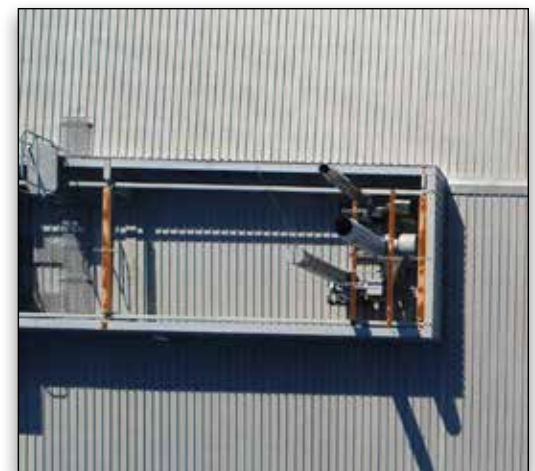
Skand projects AI-identified defects onto the ContextCapture reality mesh including forms of corrosion and building material degradation.
