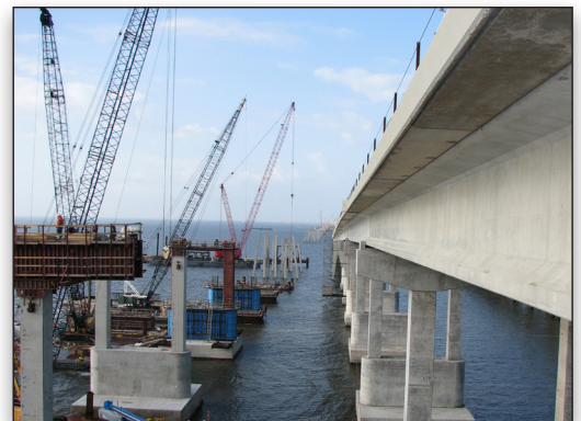
Construction proceeded at an efficient and fast pace.
