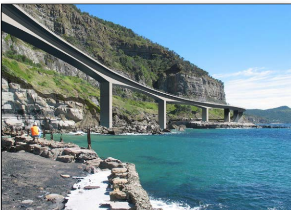
Sea Cliff Bridge on Lawrence Hargrave Drive, Australia by AECOM Maunsell Australia.
