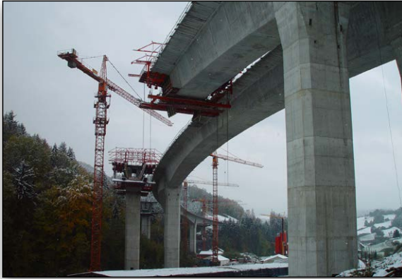
Viaduct Petelinjek, Slovenia by GRADIS, Slovenia.
